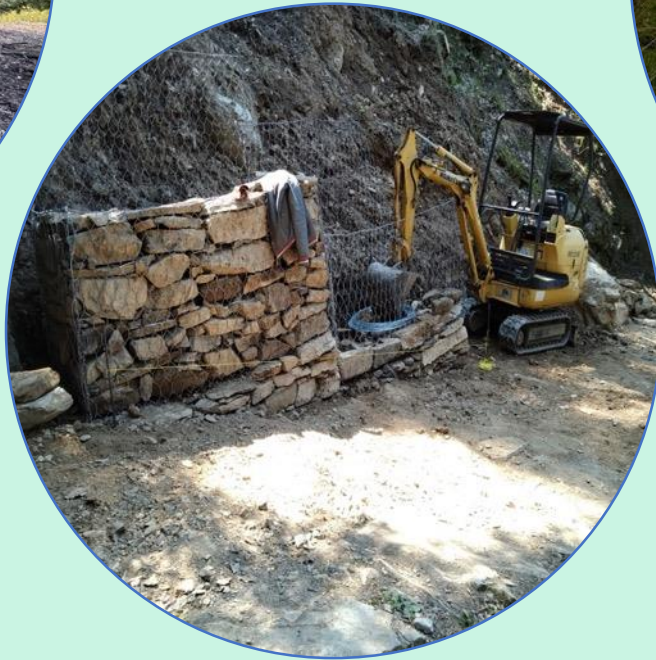
Small landslides drainage and restoration works
